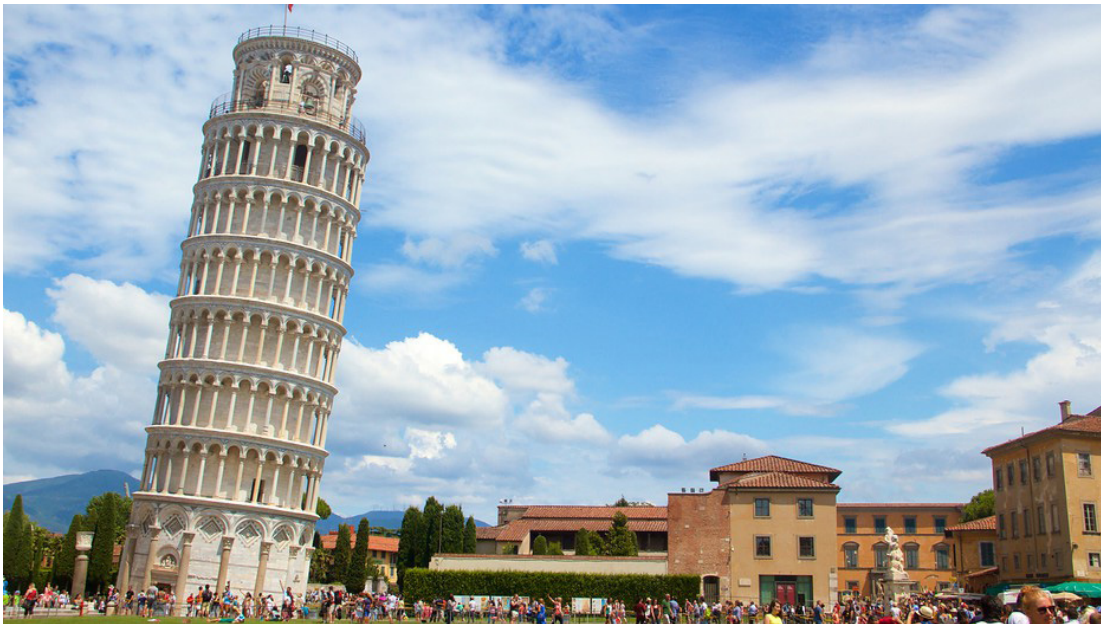
Leaning Tower of Pisa
